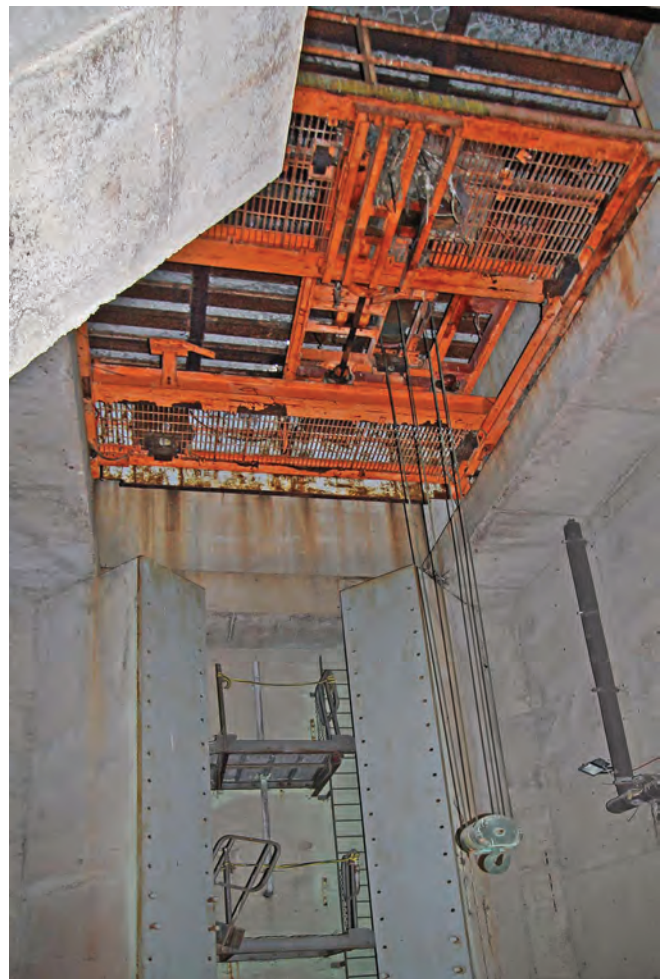
Internal view of K1. Chains and pulleys are still suspended from a gantry on the ceiling to assist in the manoeuvring of the rocket motor. At the back a ladder gives access to platforms to allow access to the motor being tested
